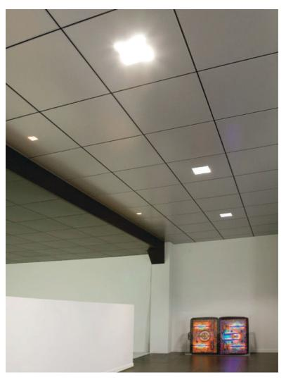
The unique shape of the profile results in a shadow joint of 8 mm on the inside of the profile. The shadow joint can be accentuated even more by using the following colour combinations:
